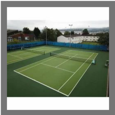
Tennis Courts Construction Services
